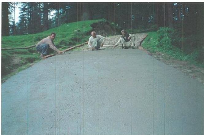
Khajjiar: Road to school being paved
