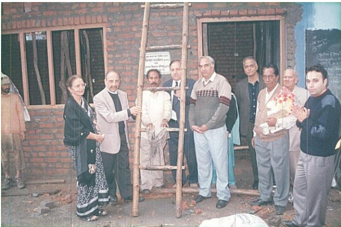
Room added to the school building - team of workers
